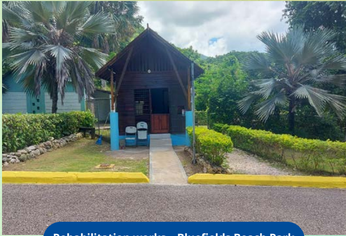
Rehabilitation works - Bluefields Beach Park
