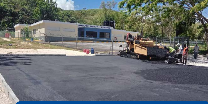
Work-in-progress - Rehabilitation of the Adelphi Health Centre Parking Area
